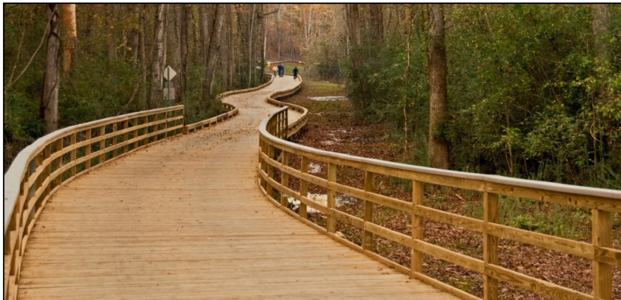
Figure 3.13.2: Big Creek Greenway Boardwalk (Source: Pond and Company, 2014)
