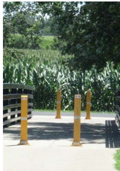
Figure 3.5.2: County Trail bridge (Source: Heartland Home Community, 2014)
