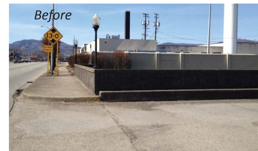
Figure 4: Existing Conditions of Gateway
