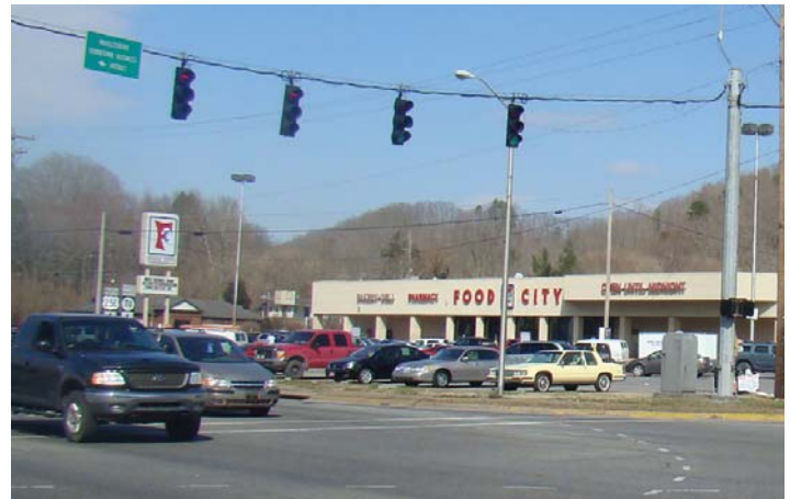
Figure 3.1.33 Existing Conditions at US 25E Intersection
