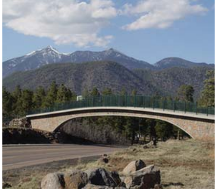
Figure 3.2.15 Matt Kelly Urban Trail Bridge (Source: City of Flagstaff, 2013)
