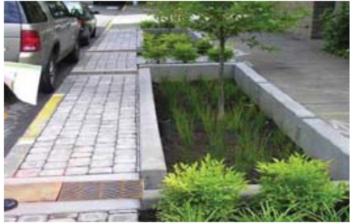
Figure 4.1.12 Storm Water Planter (Source: Smith Manage Group, 2010)
