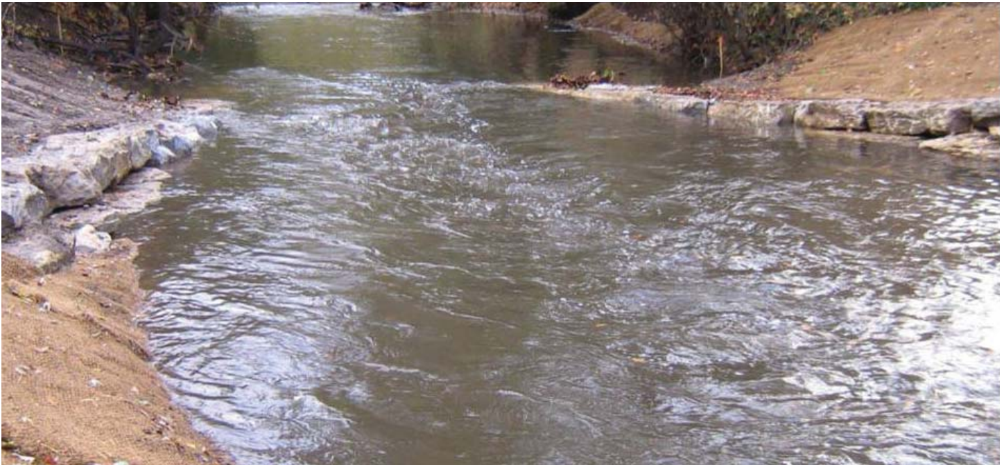
Figure 5.2.22 Cross-Vanes (Stantec, Inc., n.d.)
