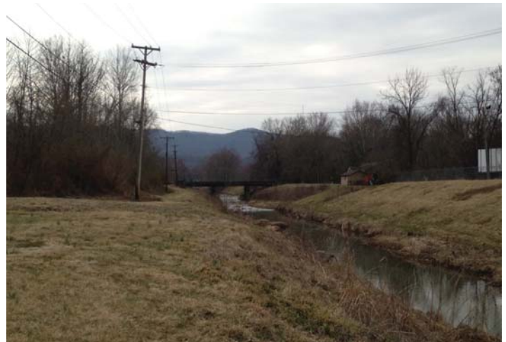
Figure 4.1.33 Existing site conditions looking towards the Sports Park
