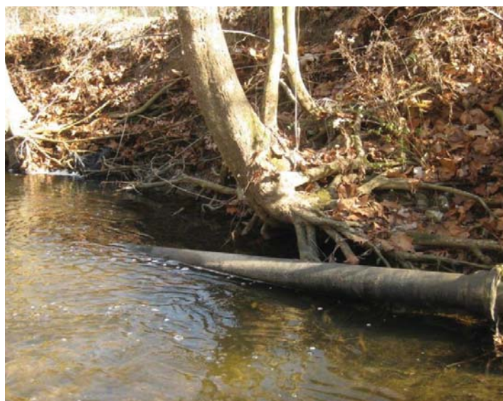
Figure 5.2.20 Exposed piping and stream pollution (Source: Stantec, Inc., n.d.)
