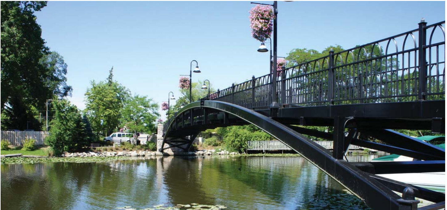
Figure 4.2.6 Pedestrian Bridge (Source: McHenry Riverwalk, 2012)
