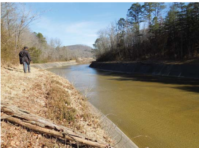
Figure 5.1.15. Existing conditions of Armored Channel
