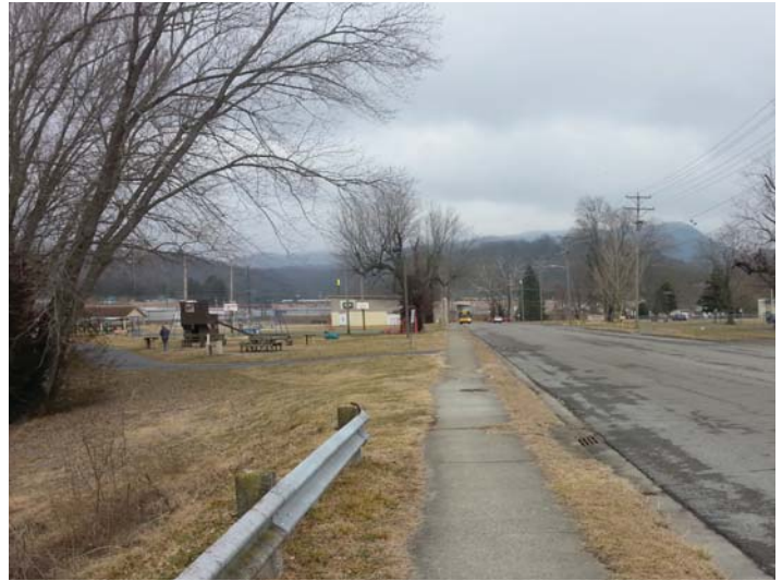
Figure 4.1.24 Current condition of Lothbury Avenue
