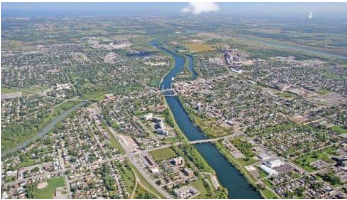
Figure 4.2.21 Waterway Aerial (Source: Welland Recreational Canal Corporation, n.d)
